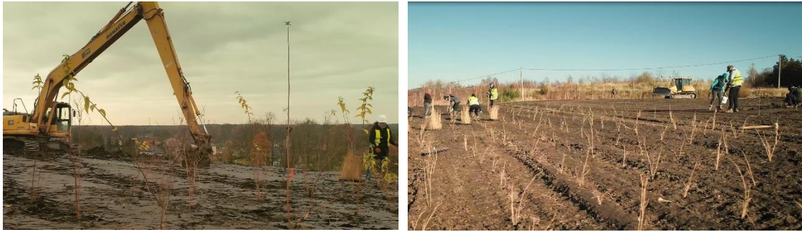
Figure 9 – Polygon test construction
