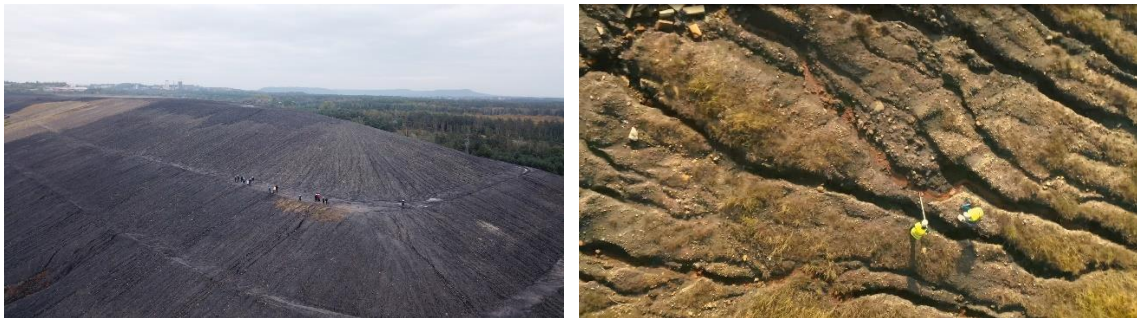
Figure 7 – Libiąż waste heap and the erosion slopes
