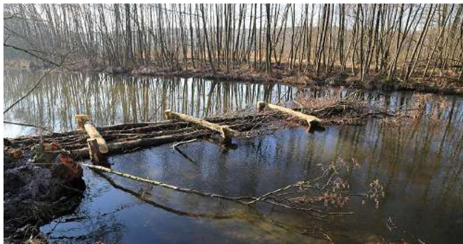
Fig. 1 Groyne made of dead wood to encourage re-meandering
