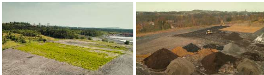
Fig. 1 Land rehabilitation at Libiąż coal waste heap in Poland
