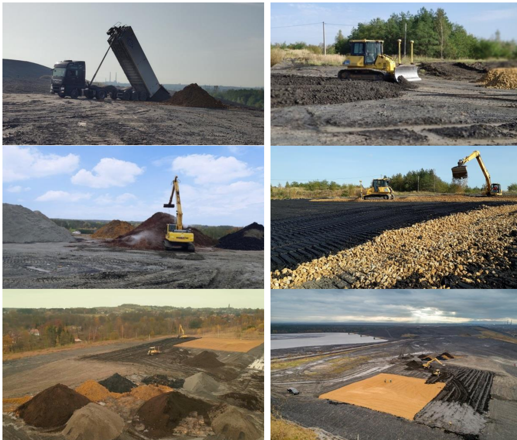
Figure 17 Field works on the Janina waste heap
