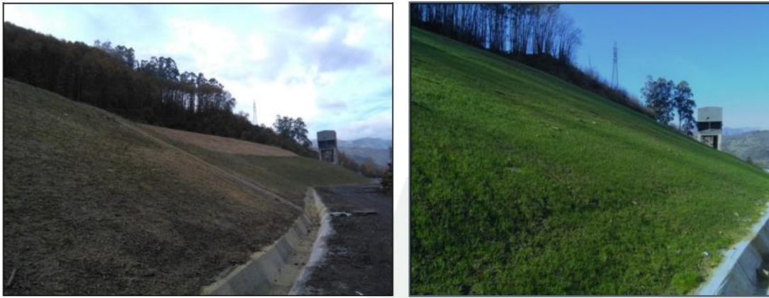
Figure 11. Hydroseeding results after six months in Sector 2 (Nov. 2016 – May 2017)
